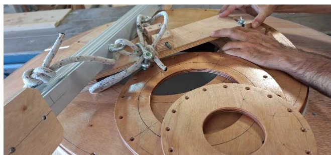
Figure 8: Construction process of the conical dome made from ply wood
